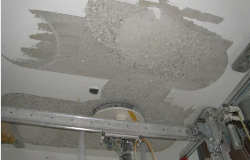
Wall shaver during shaving the ceiling in the powder room
