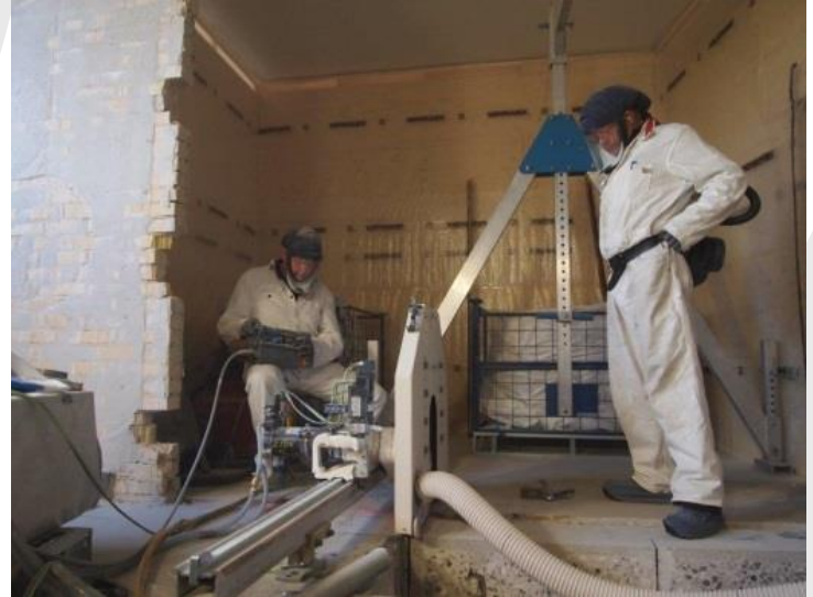
Sawing of the floor in the powder room
